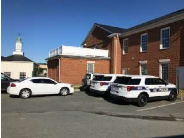
Figure 2. The town's police department is located in Town Hall (staff photo, 2017).
