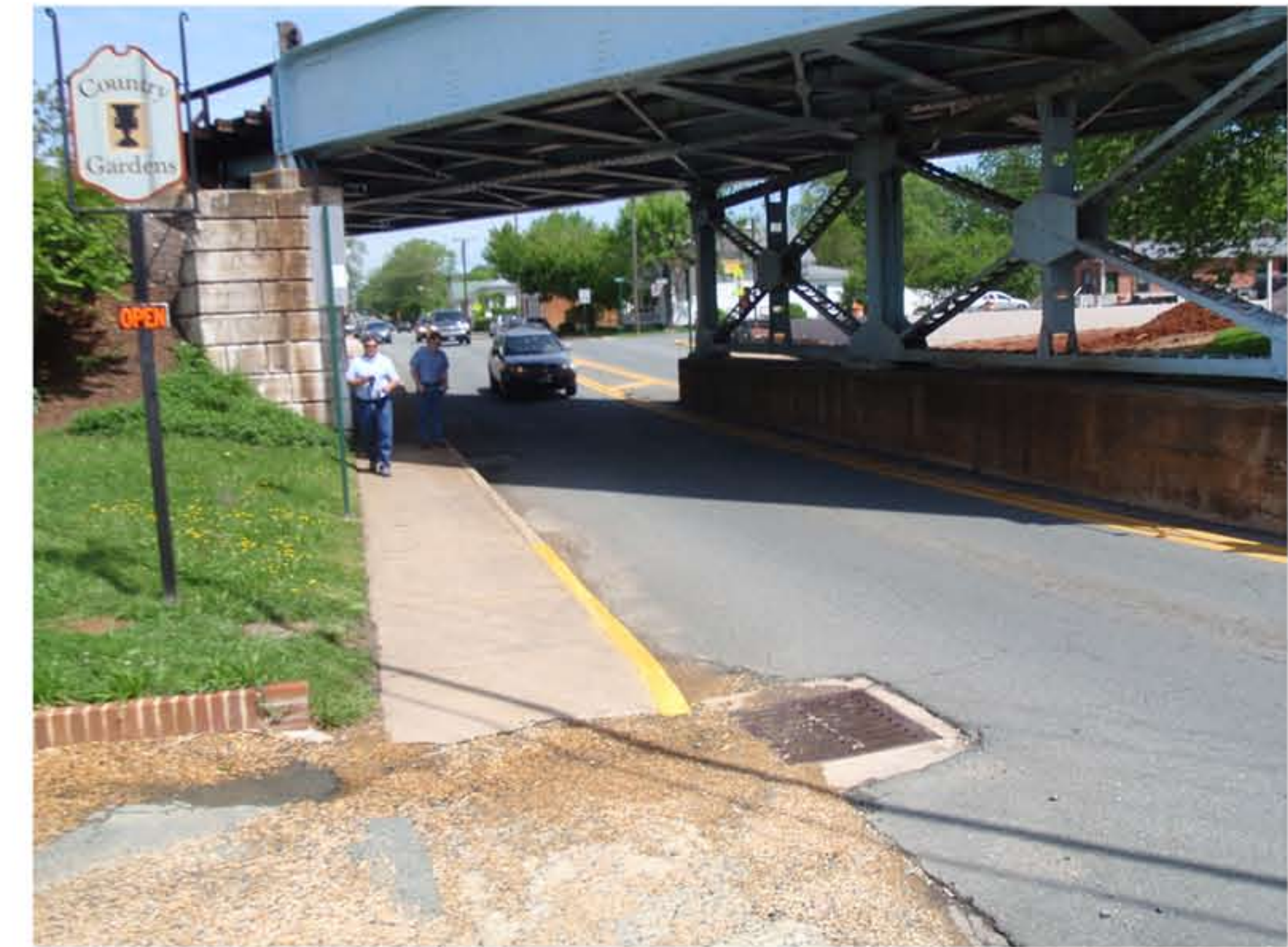
Rail Road Underpass
