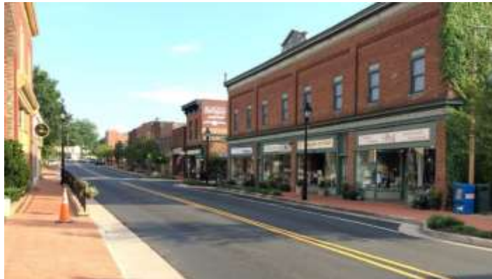
Figure 2. Businesses line Main Street in Downtown (staff photo, 2016).
