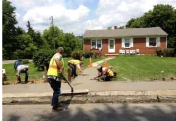
Figure 3. Town Crew works to construct the East Street sidewalk (staff photo, 2013).
