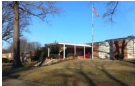
Figure 6. Gordon Barbour Elementary School (staff photo).
