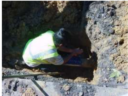
Figure 1. A member of Town crew works to repair a water leak on South Main Street (photo by Town staff).
