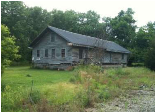
Figure 9. The Freight Depot (staff photo, 2013).
