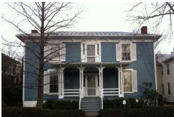
Figure 11. The E. J. Faulconer House on Main Street (staff photo, 2013).
